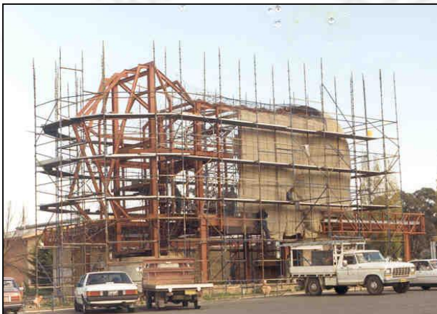
Structural Steel Framework Merino Ram - Goulburn - Australia
